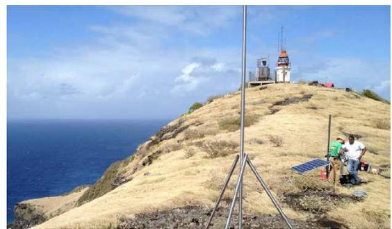
Partially installed GPS monument for site NC47. UNAVCO field engineers worked with faculty and students from the University of the West Indies Seismic Center on the installation. Photo credit: J. Sklar
